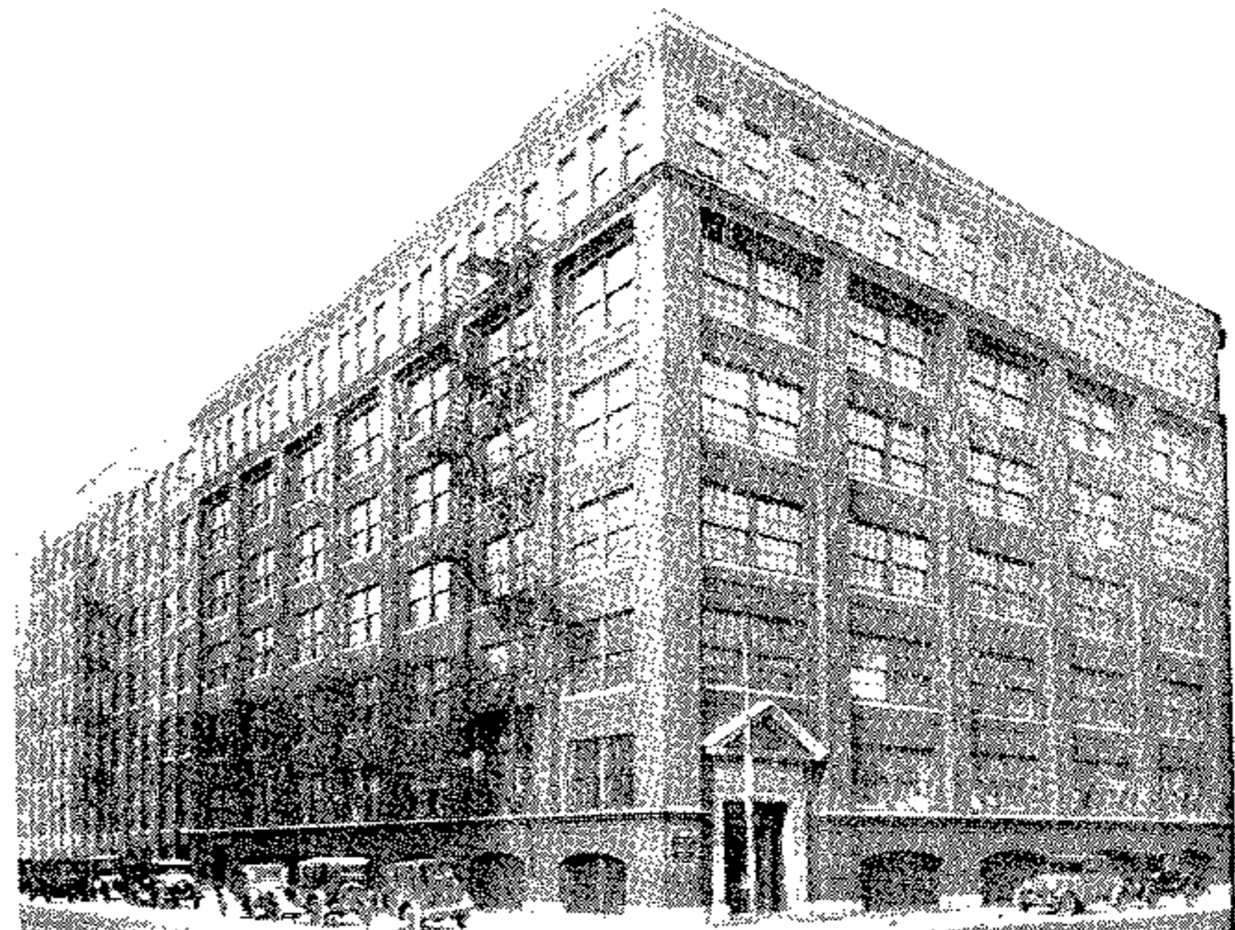
The THORDARSON Factory—the largest plant in the world devoted exclusively to the manufacture of transformers.
